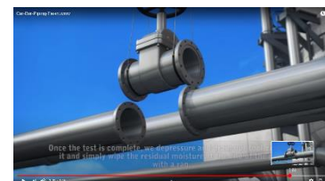
Step 13 (Prepare flange ends for joint fit-up)
