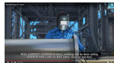
Step 9 (Inert gas purging & welding of flange)
