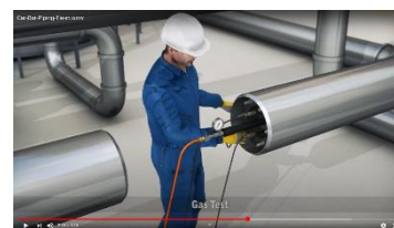
Step 8 (Isolate and perform gas test)
